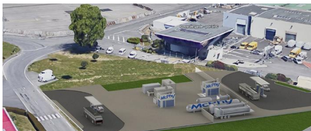
Figure 2: Station Hydrogène ATB [11].
